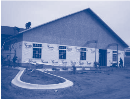
Progress — O'Harrow Construction works at North St.
